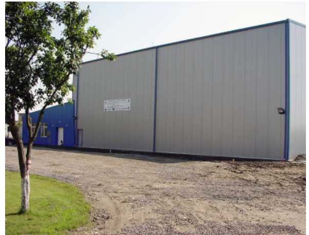
Fig. 1. Office complex with attached building for hydrotechnics system. © Hydro-Elektrik GmbH
